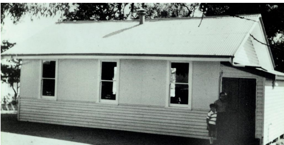
(The Graylands State School after renovation - 1940)
